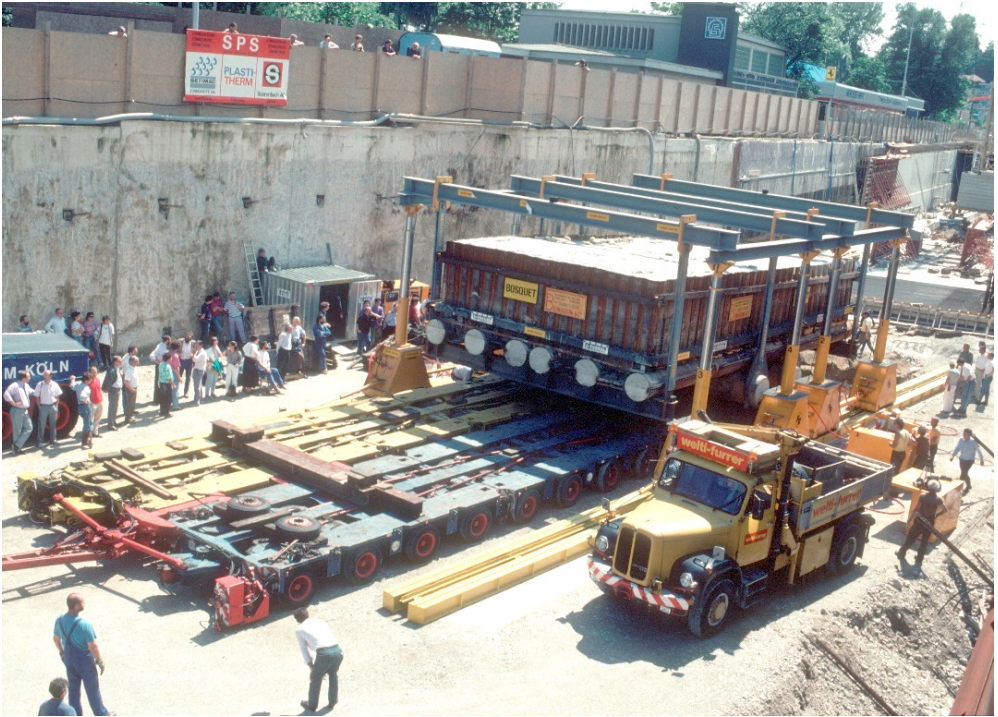
Fig. 4: Motorway excavations have been the framework of large scale preventive operations. Here the removal of a part of the archaeological site of Monruz (NE) during the construction of the Motorway A5 in 1991 (Photography: Béat Arnold, Laténium).
