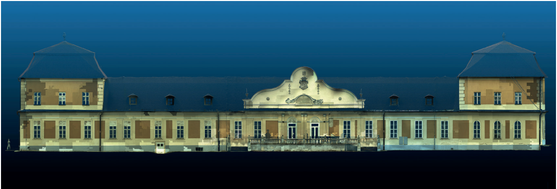
Figure 5. Manor house at Žehra, Hodkovce, Slovakia. Point cloud with RGB values showing exposure inconsistency due to poorly exposed composite photos taken by the native scanner camera (Leica C10).
