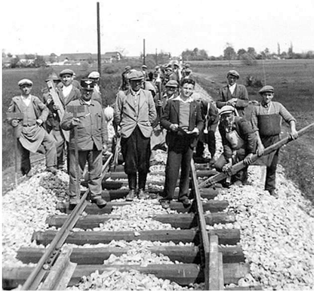
Fig. 9: Laying railway tracks near Hodoš in 1941.
