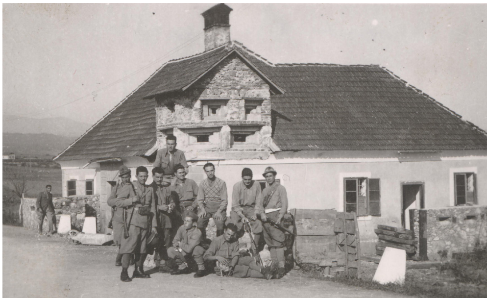
Fig. 4: The Italian Army converted a house near the bridge across the river Kolpa near Metlika into a bunker.
