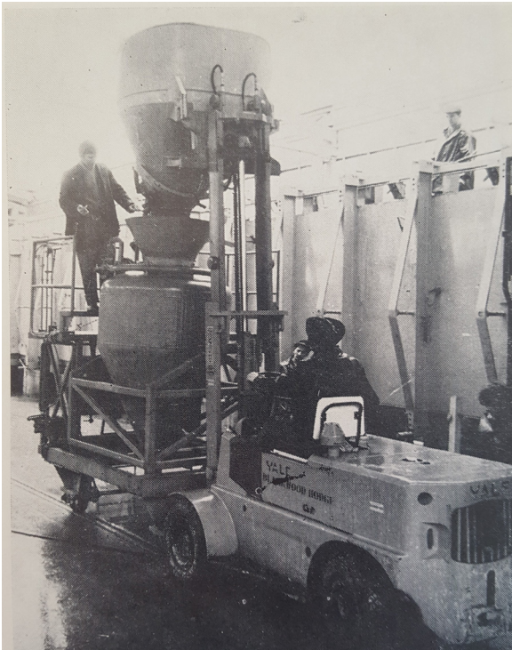
Figure 8: Close up of concreting plant and moulds for vertical casting. Concrete is injected from the bottom of the mould (Cubitts Haden Sisk: Ballymun housing project, 1966).
