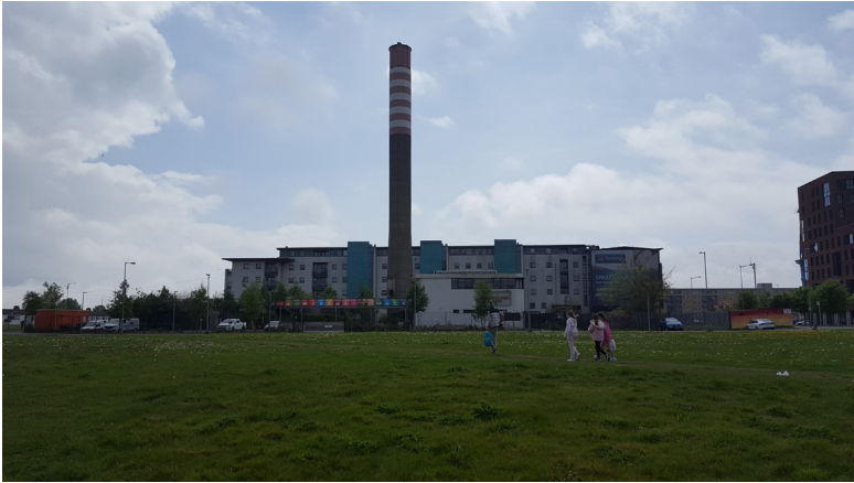
Figure 20: Old boiler house building from afar. Photo: Alina Bezljaj, 5/7/2022.
