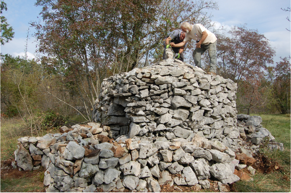
Figure 3: Boris Čok and Dušan Okoren finishing the roof of biška , 2014 (Eda Belingar).
