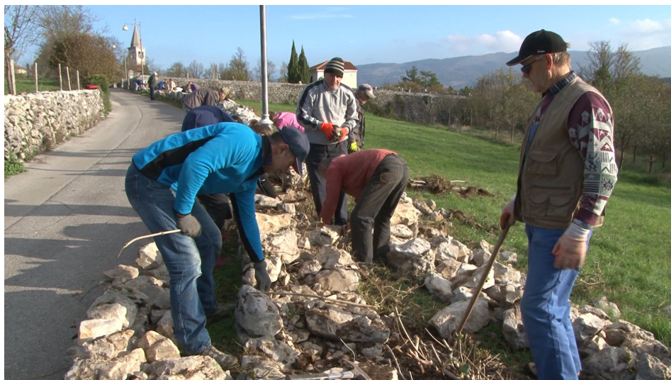
Figure 8: The dry stone wall was dismantled, Škocjan, 2016 (image from Dry Stone Walling , Nadja Valentinčič Furlan).
