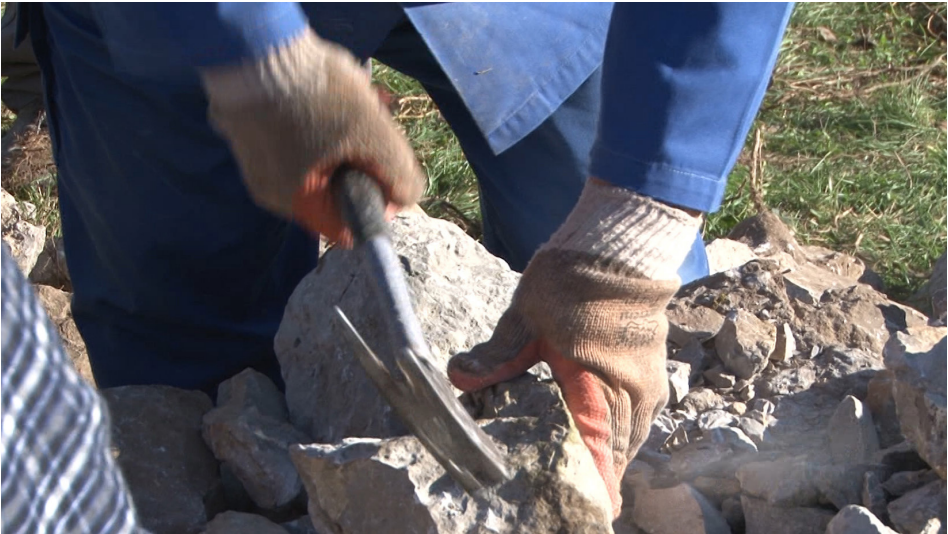
Figure 11: Cutting the edges of the stone to make it fit into the wall, Škocjan, 2016 (image from Dry Stone Walling , Nadja Valentinčič Furlan).
