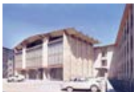
Administrative building of the District People's Committee (OLO) of Kranj, Kranj (as Edvard Ravnikar's collaborator), 1955
