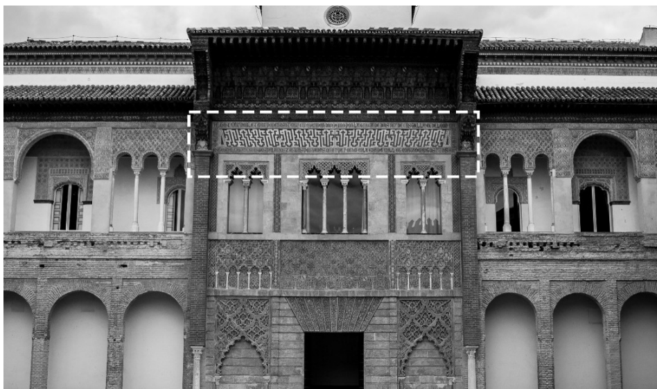
Figure 10. Façade of the Palacio de Pedro I , Alcázar of Seville. The architectural programme demonstrates the strategic appropriation of Islamic visual codes by Christian monarchs to consolidate authority. Notably, the Gothic script – detailing that the “The very high and very noble and very powerful and very conquering Don Pedro, by the grace of God king of Castile and Leon, ordered to be made these fortresses and these palaces and these gates which were made in the year one thousand and four hundred and two” 29 – is positioned directly above the Nasrid motto, Wa-lā gālība illā Allāh (“There is no conqueror but God”).
